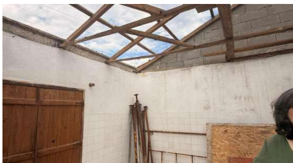
Before the intervention
